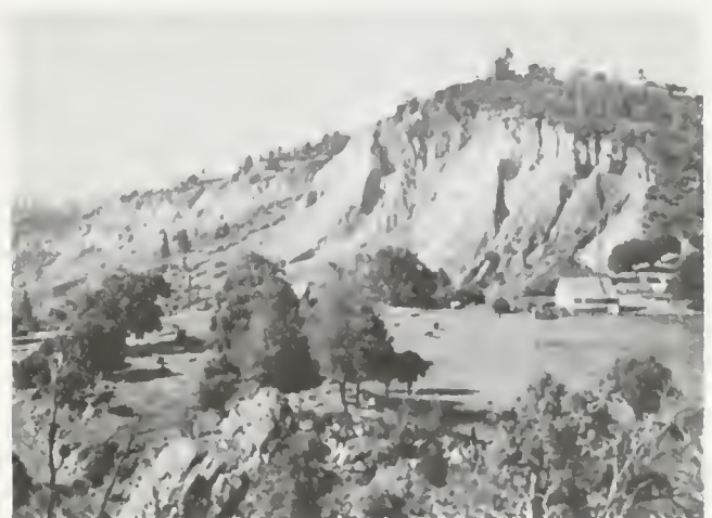
Figure 26. West face of Cherokee hydraulic mine, with outcropping bedrock in foreground. View south from Cherokee.
